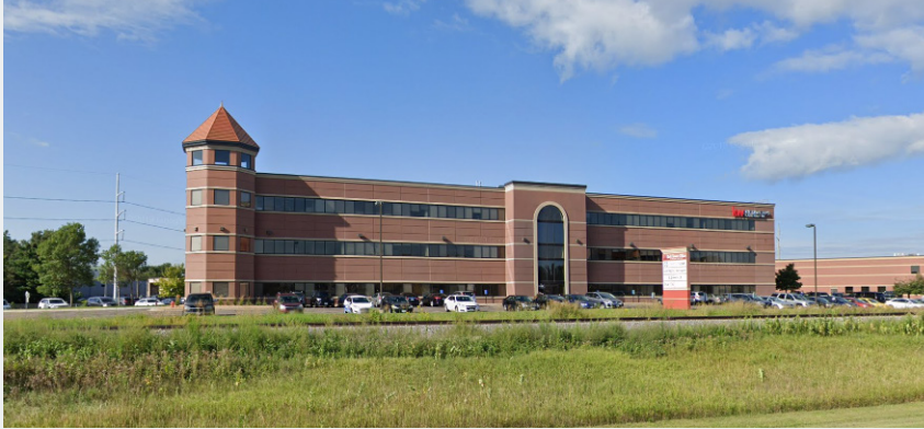
Front of Building
