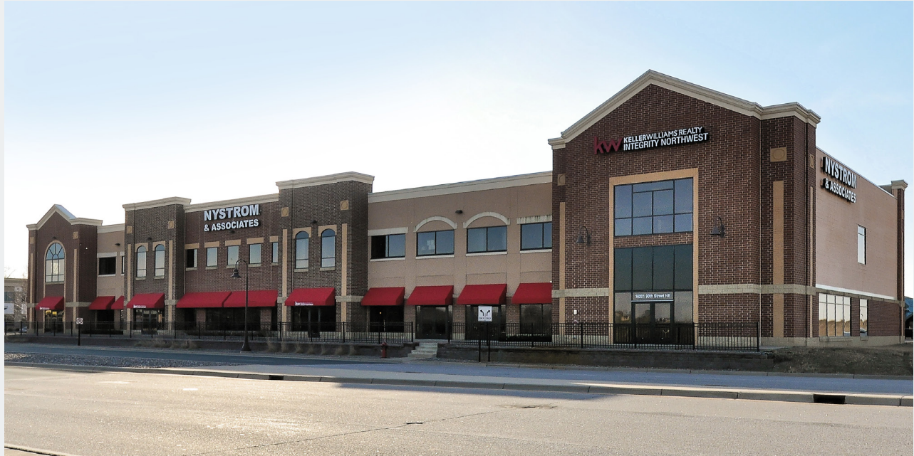
Front of Building
