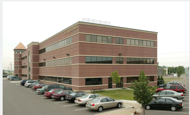
Front of Building
