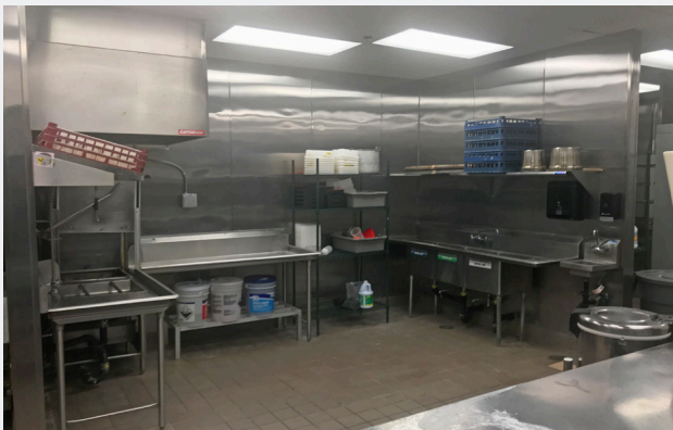
Restroom Kitchen View
