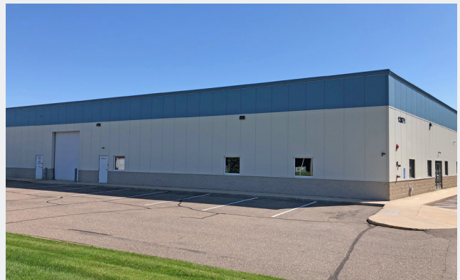
Drive in door/entry
